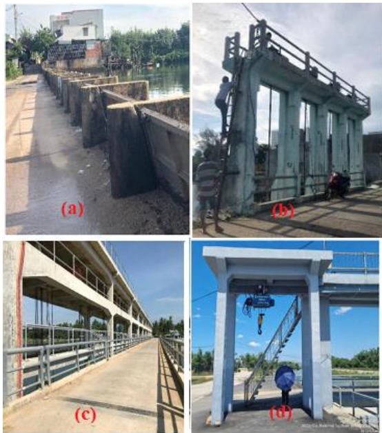
Figure 1. The manual lifting and lowering operating mechanism is through a Vitme.
