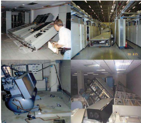
Figure 1. Damage of non-structural components. 19
