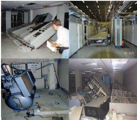
Figure 1. Damage of non-structural components. 19
