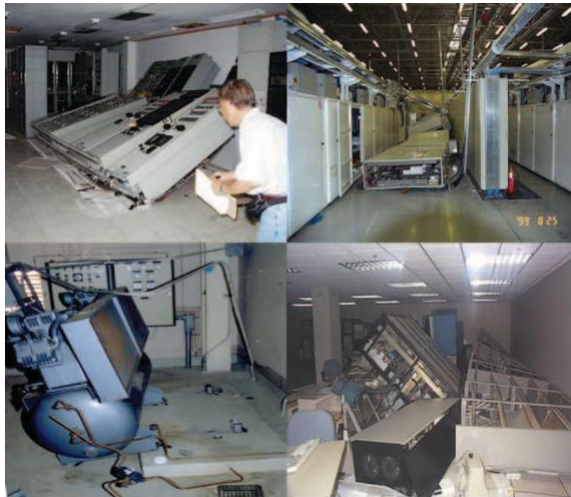
Figure 1. Damage of non-structural components. 19
